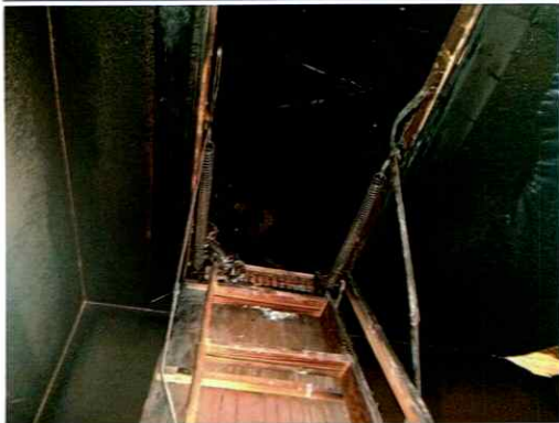
56-Front Room Attic
